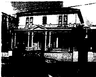
215 VIVIAN STREET Part Relocation, Part Demolition – rear portion of building
